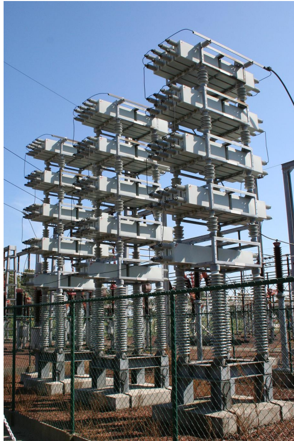
Figure 58 75MVAR substation capacitor bank at 150kV
