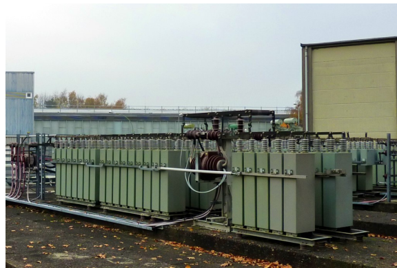
Figure 57 One of several energy storage power film capacitor banks, for magnetic field generation at the Hadron-Electron Ring Accelerator (HERA a ), located on the DESY b site in Hamburg c
