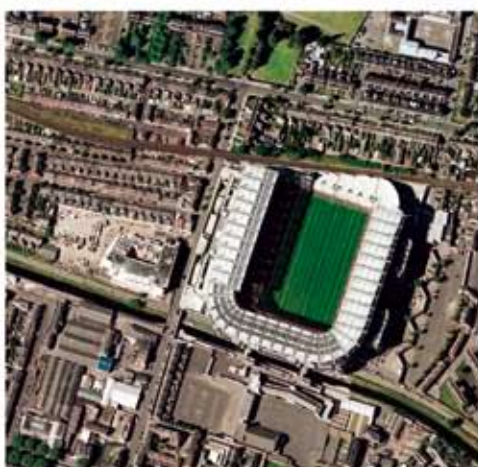
Image courtesy of BKS Surveys Ltd.
