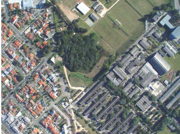
Figure 1: Aerial image taken with Sony camera employed in this research.
