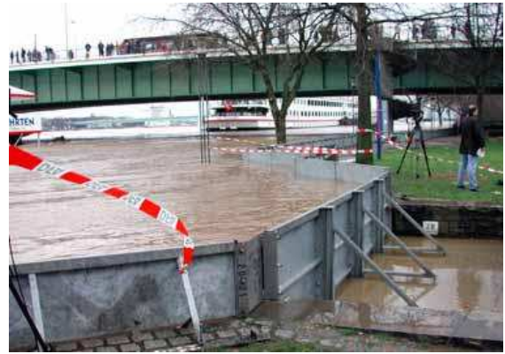
Figure 7: Mobile wall in the city of Cologne †
