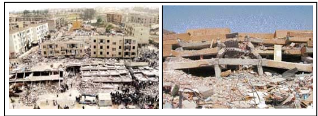
Figure 7 Building damage in Boumerdes (courtesy of AP Photo and EERI)
