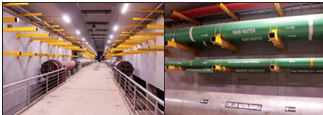
Fig. 3: Utility Tunnel in GIFT City, District Cooling System (DCS)
